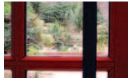
Figure 4.13 Objects or areas of glazing which could be obstacles for the visually impaired or older people should contrast well with backgrounds
