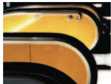
Figure 4.39 Coloured escalator side-panels can be functional for accessibility, wayfinding and yet be part of a lively colour scheme
