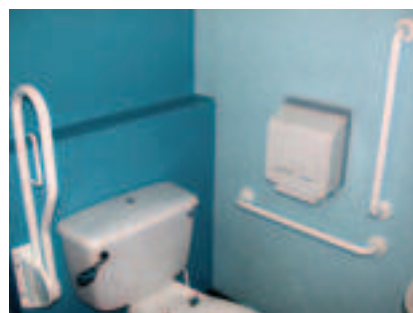
Figure 4.28 Contrasting walls from sanitary ware is helpful for the older or visually impaired to use wash-room facilities with confidence
