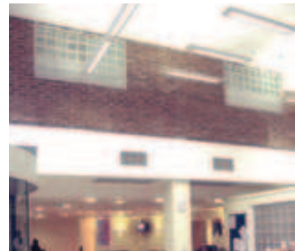
Figure 3.11 In this day-lit entrance, high level suspended fluorescent fittings brighten the ceiling on dull days. Their cool colour complements that of daylight, contrasting with the cosier, warmer coloured lamps in the adjacent waiting area
