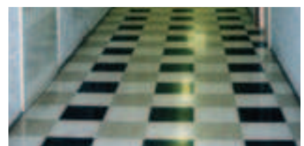
Figure 2.62 Simple designs in flooring work best. Try not to use too dominant a geometric design which can cause disorientation for some people
