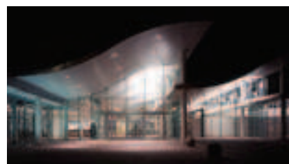
Figure 4.10 The foyer of the hospital should look welcoming from the outside by day and night
