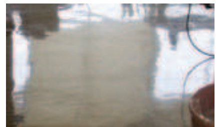
Figure 2.60 Glossy floors cause major glare problems for elderly and visually impaired people. Alternative surfaces should be used
