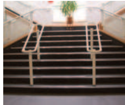
Figure 2.2 Use of contrast and tonal detail for accessibility is provided by a colour design guidance strategy
