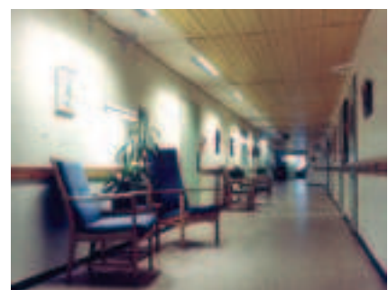
Figure 4.46 Illuminated vertical surfaces and offset luminaires used to light a corridor space
