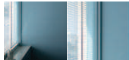
Figure 4.58 Blinds can soften strong daylight and direct light further into the room
