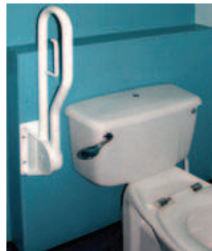
Figure 4.73 Toilet facilities can be part of colour schemes used throughout a ward. Using a contrast colour behind sanitaryware aids older and visually impaired people. A complementary colour from the harmony schemes would provide visual interest by a change from the ward colour schemes. This would be beneficial for long-stay patients
