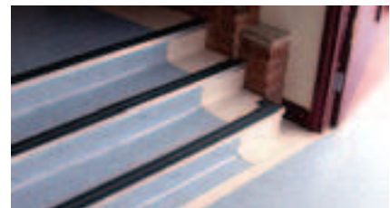
Figure 4.38 Colour contrast seen on approaching stairs and nosings help visually impaired people
