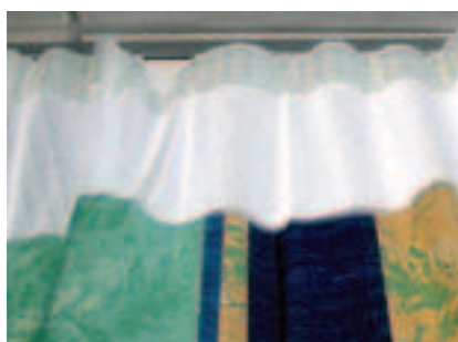
Figure 2.83 Translucent panels at the top of these curtains provides some filtered light into a bed area within a maternity unit preserving privacy without excluding daylight
