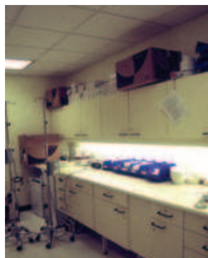
Figure 3.14 Lighting under the cupboards gives excellent glare-free task lighting in this drug-dispensing area. The standard ceiling lighting would not have been sufficient on its own, as the light to the task would have been shielded by the staff themselves
