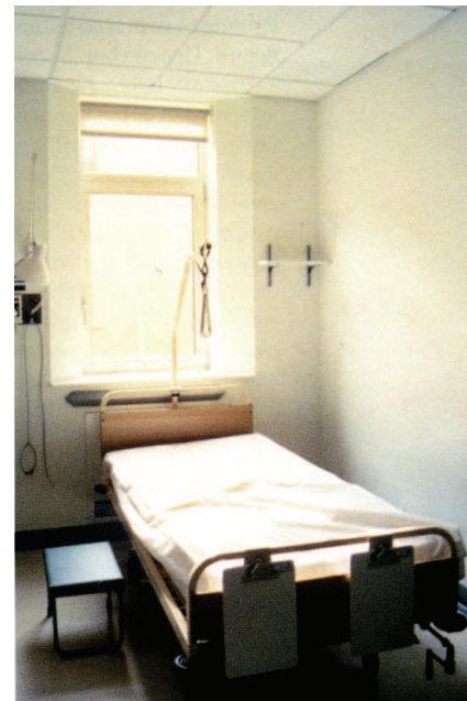
Figure 3.7 Splayed reveals surrounding windows can control sky glare by reducing the contrast between window and wall
