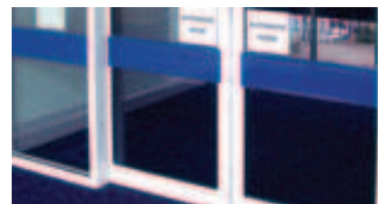
Figure 4.6 Glass doors require adequate manifestations to alert people approaching glazed panels or doors from a reasonable distance
