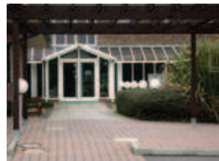
Figure 1.8 An external entrance to a children's unit is scaled down for a child's perspective. External illumination has been reduced in height
