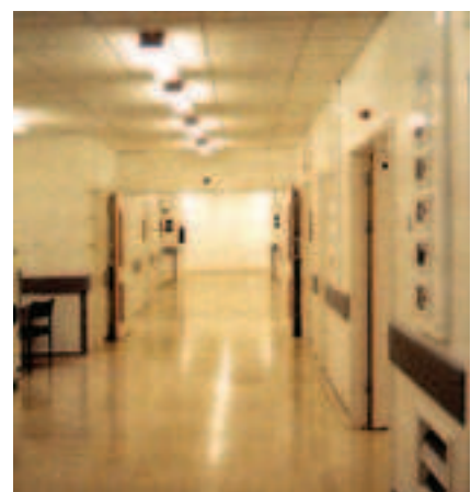
Figure 4.45 Shiny polished floors create glare when illuminated with artificial lighting
