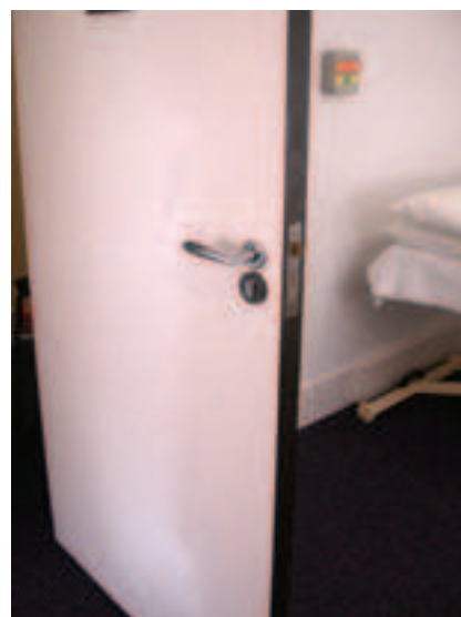
Figure 1.6 Use of strong contrast on potential obstacles, such as edges of doors, aids safety and accessibility for all
