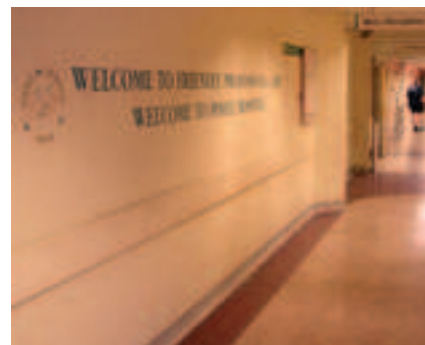
Figure 4.49 Floor boundary colours created for wayfinding helped reduce wall damage from straying trolleys
