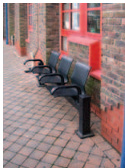
Figure 2.6 Potential obstacles such as seating which might be dangerous should be finished in contrasting colours
