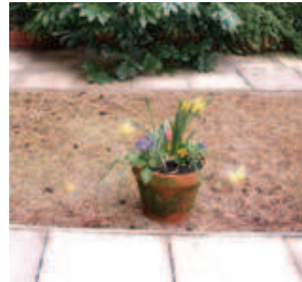
Figure 2.14 Light-coloured aggregate or paving material on surrounding pathways can enhance levels of reflected light back into the building interior
